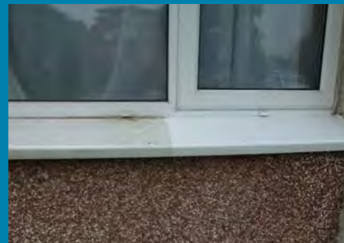
UPVC BEFORE AND AFTER ▲
