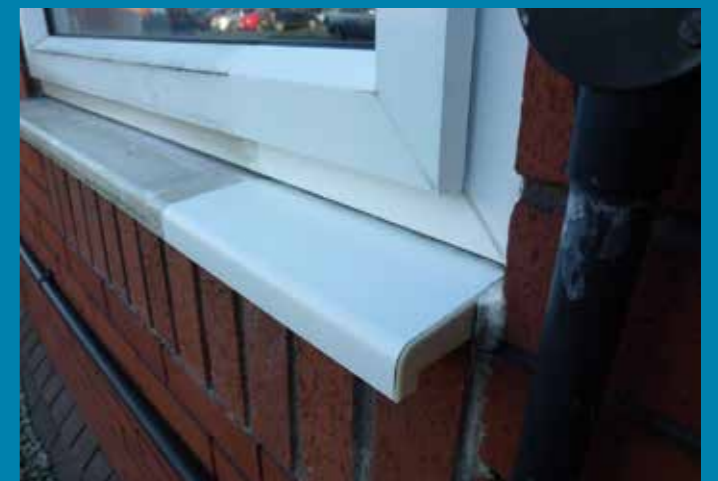
UPVC BEFORE AND AFTER ▲
