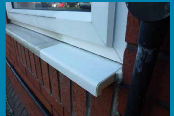
UPVC BEFORE AND AFTER ▲
